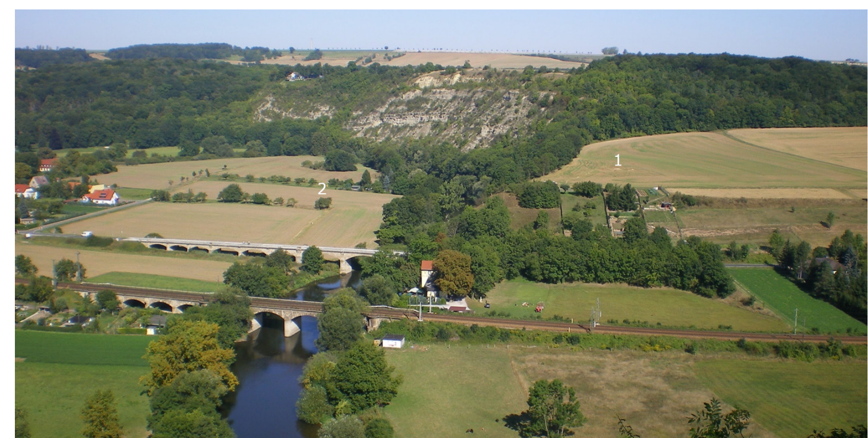
Fig. 2: View of the site from the south, taken from the tower of Saaleck Castle. 1: Bad Kösen-Lengefeld, 2: Saaleck.
