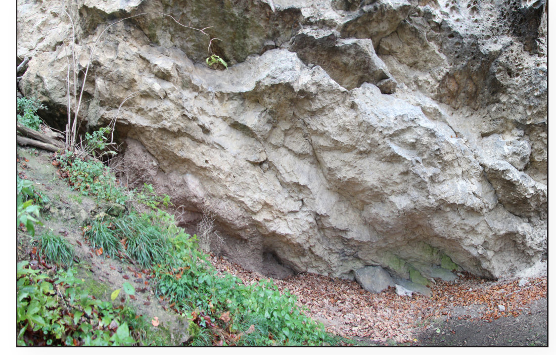
Fig. 10: The rockface at the planned excavation area. In the highlighted area, solidified sediments are still clinging to the wall.
